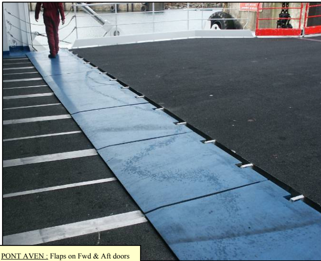
PONT AVEN: Flaps on Fwd & Aft doors
